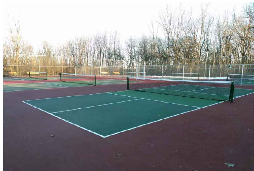
EXISTING CONDITION GARNER PARK PICKLEBALL COURTS
