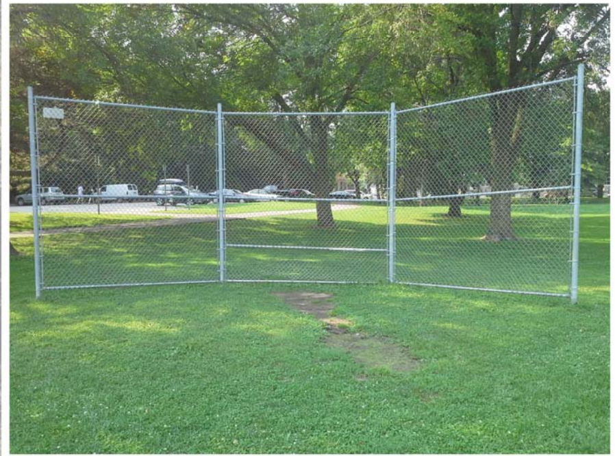
EXISTING CONDITION WINGRA PARK BACKSTOP
