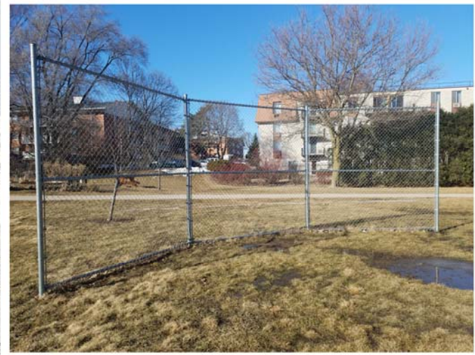
EXISTING CONDITION RENNEBOHM PARK BACKSTOP
