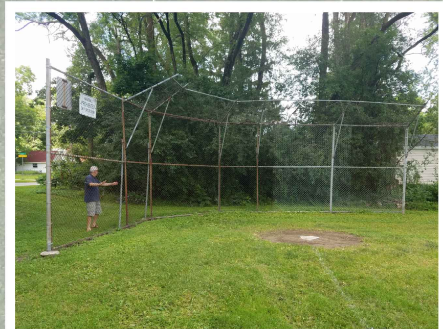
EXISTING CONDITION - BORDNER BACKSTOP
